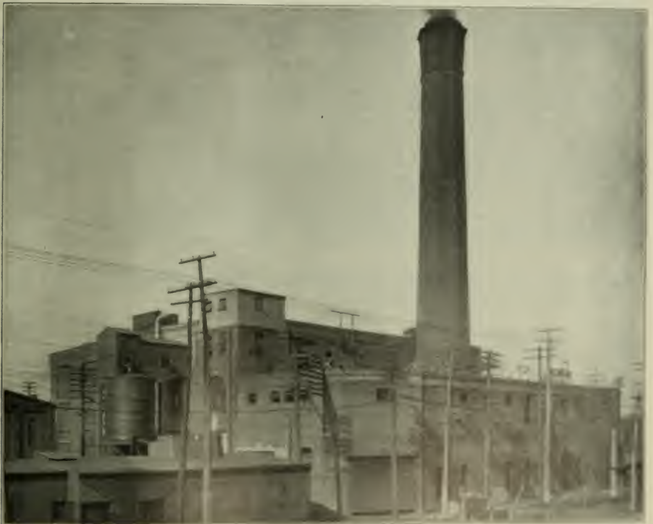
FIG. 1. EXTENSION OF FOURTEENTH STREET POWER STATION, LOUISVILLE, KY.
